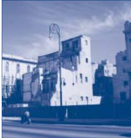
As buildings are renovated, most façades survive, but some are in such poor structural condition that they are lost and will need to be recreated from scratch.
