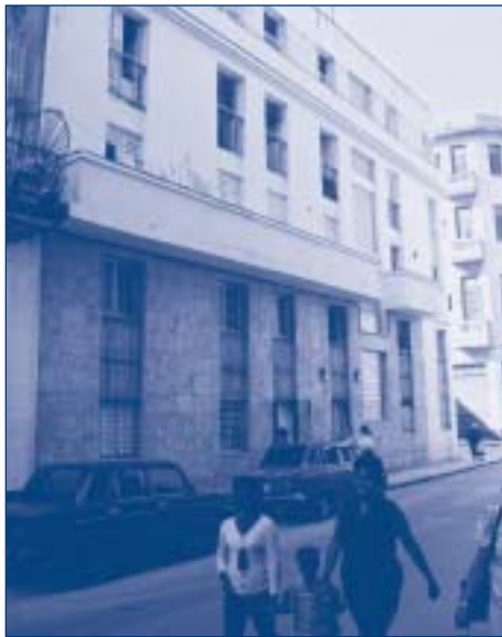
A few blocks inland at the corner of Crespo and Refugio streets, a new apartment building for temporary placement of residents of buildings under renovation.
